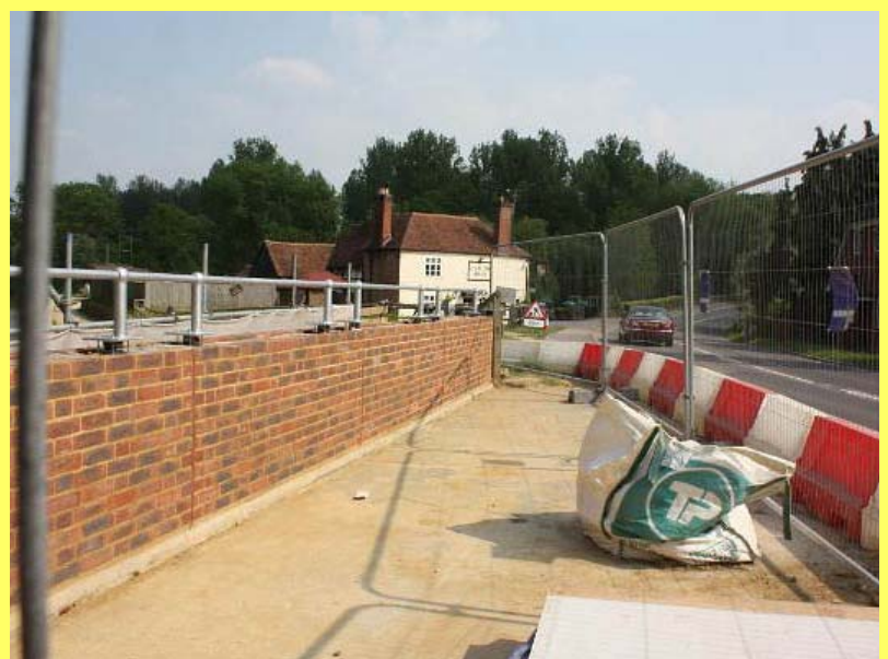
The new parapets take shape at Loxwood (Richard Crook)
