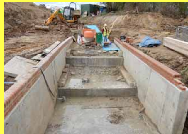
Northern working party making good progress on the summit level slipway (Bill Nicholson)
