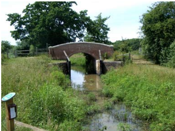
The flood gates at Lordings, south of Billingshurst, accessible via the Wey-South Path
