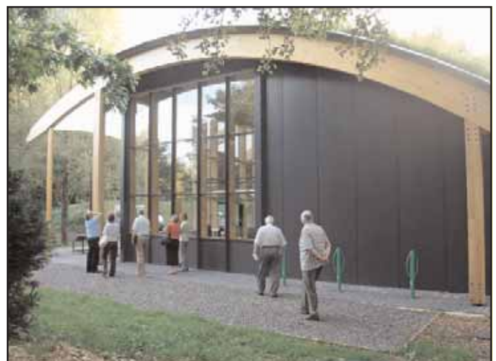
The Greenpower building at Fontwell - WACT's visitor centre will be a much smaller version of this (Bill Thomson)
