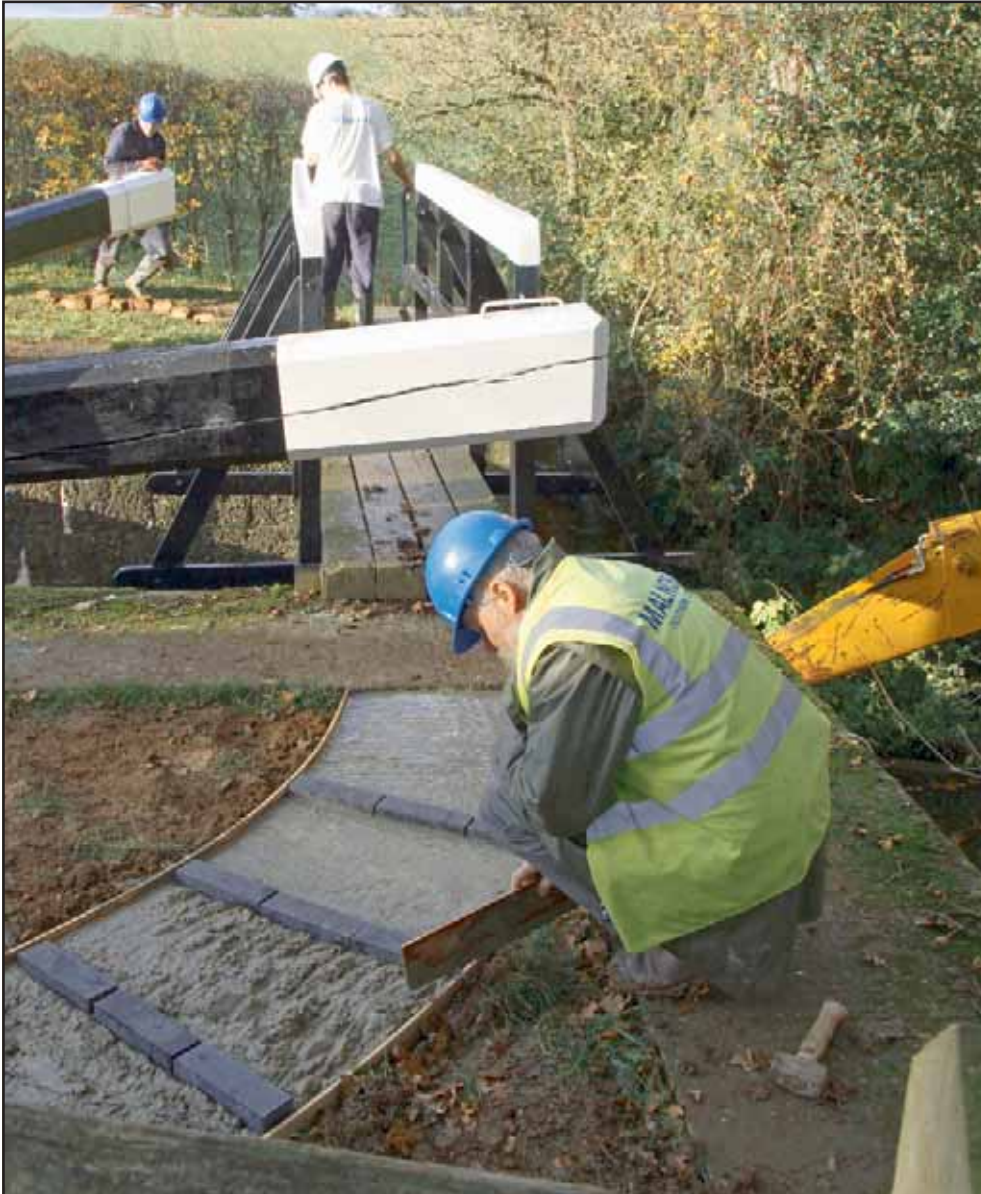
Installation of new quadrants by the NWPG weekend campers (Julian Morgan)
