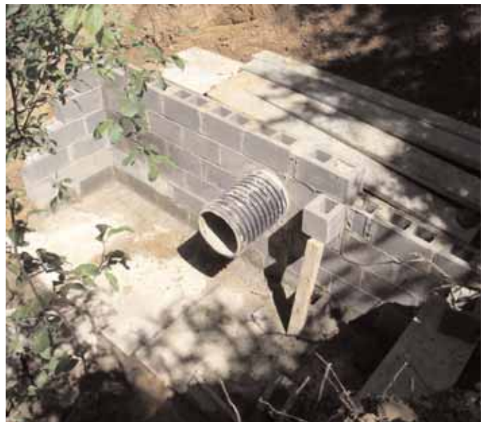
The new culvert south of Southland Lock, the TSG's current project
