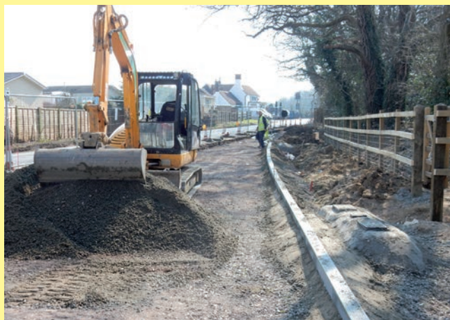
Preparing the carriageway at Compasses Bridge
