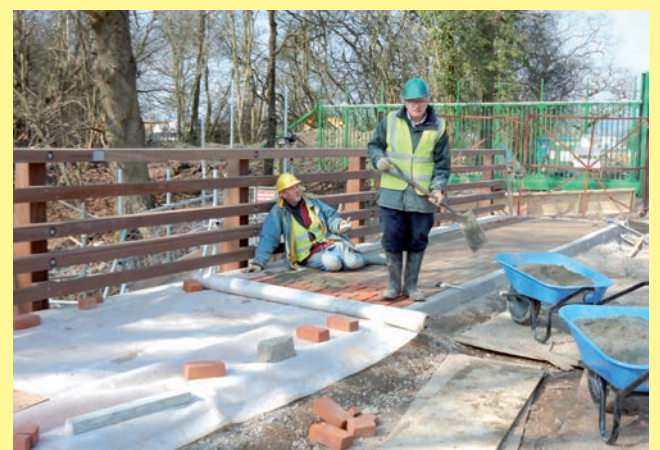
Paving the southern footway at Compasses Bridge
